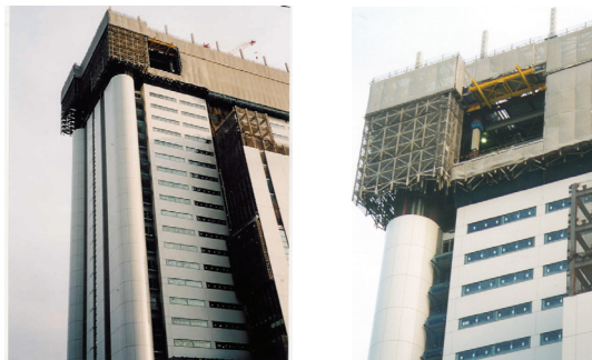
Fig. 1. An automated construction system in Japan.
